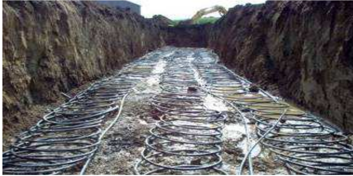
Figure 6.18: Horizontal Ground Source Heat Pump Loop
